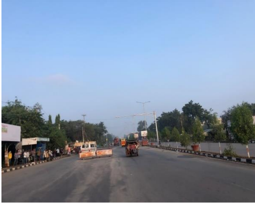
Fig.19: At chainage 7.100 Km, in this picture barricades are provided to slow the traffic and to provide bus transportation for passengers at the stop.
