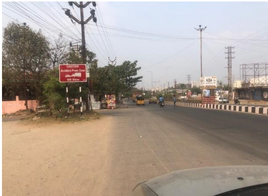
Fig.5: At chainage 1.400Km, Accident prone Area sign board: A sign board indicating the area as accident spot and advising the vehicles to travel with low speed on a specified road. But road markings are not present.
