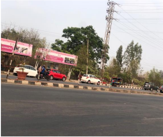
Fig.20: At chainage 7.400 Km, Unauthorized parking by group of vehicles along the road.
