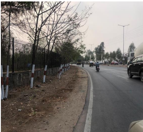
Fig.18: At chainage 6.600 Km, no sign board is maintained indicating left turn which increases the risk for vehicles.
