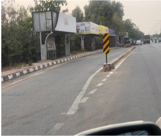
Fig.16: At chainage 5,900 Km, Bus Bay Junction Lane was separated from normal traffic.
