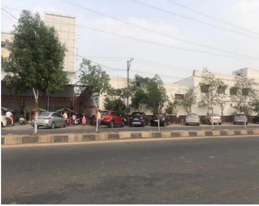
Fig.13: At chainage 3.900Km, Accident might happen due to parking of cars on the roadside. (Ice cream factory named as ... Employment generator or trip attraction centre. However inadequate parking for the customers forcing them to park vehicles on the SH.
