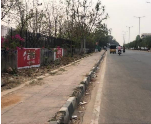
Fig.4: At chainage 0.800km, footpath of 3km length and width 1.3m is provided for pedestrians.
