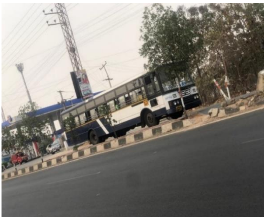
Fig.15: At chainage 5.700 Km, Unauthorized gap in median is made by people traveling towards petrol bunk.
