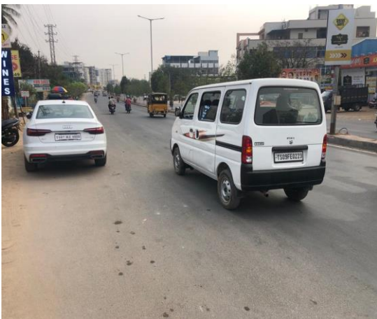
Fig.9: At chainage 2.300Km, there is no shoulder for car parking. The vehicles are parked on side of a road. Adequate enforcement shall be applied to restrict parking in no-parking zones.
