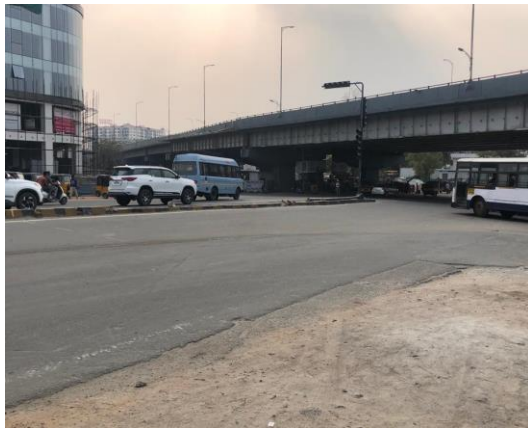
Fig.26: Chainage (15.000 Km) Sagar Ring Road junction which is at the end of Stretch, major junction without proper functioning of traffic signals. The traffic from flyover converging in to Junction without a traffic signal is a major spot for accidents happening over there.
