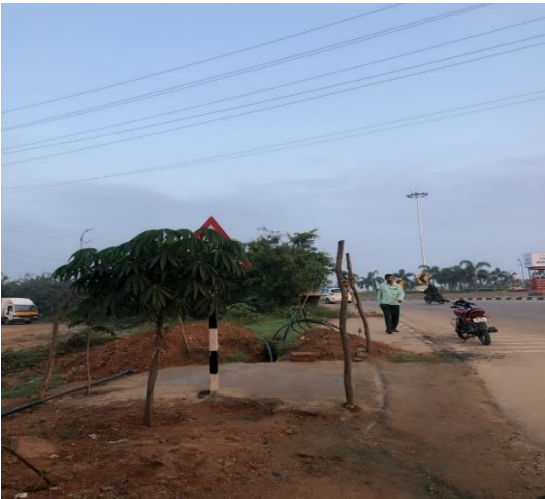
Fig.8: At chainage 1.900 km, Roundabout ahead sign is blocked by vegetation beside the road. And poor visibility signs at CH:3.600 km, 6.800 km, 9.000 km.
