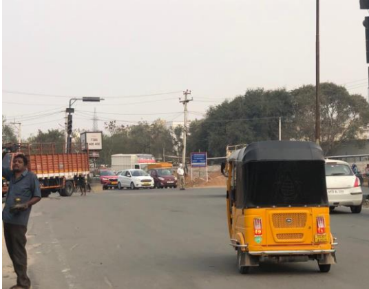
Fig.25: Chainage 14.700 Km, have a Junction without working traffic signal. Junction with considerable amount of traffic without a working traffic signal is a major spot for accidents.
