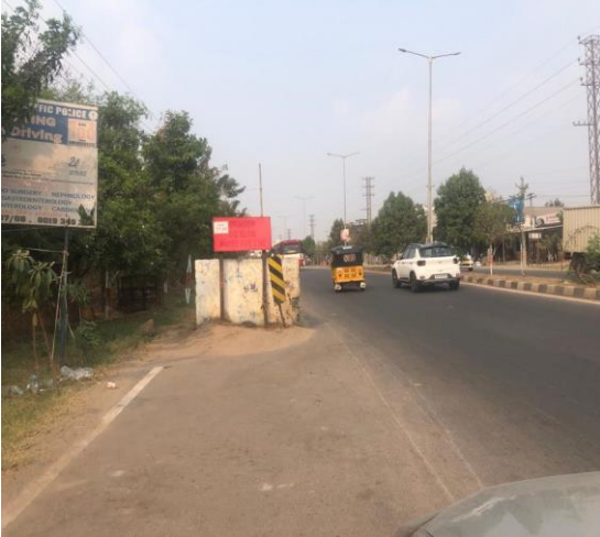
Fig.7: At chainage 1.600Km, Due to construction of a water pipeline, bottle neck condition is formed causing traffic.
