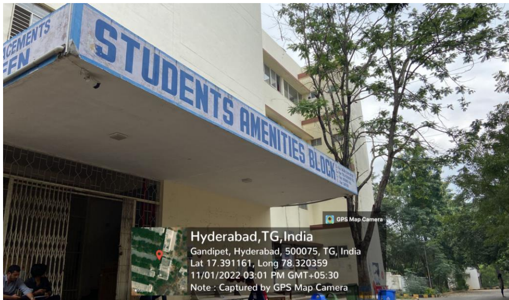
CC TV cameras are installed at the entrance of the canteen
