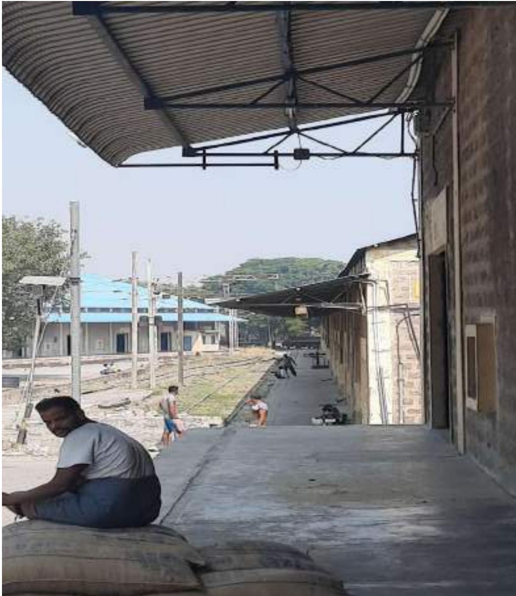
Fig: Railway platform for wagon loading and unloading
