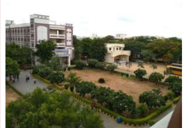
EEE department Front View
