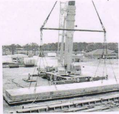
Rail containment slab
