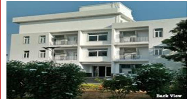
R&E Hub Back View
