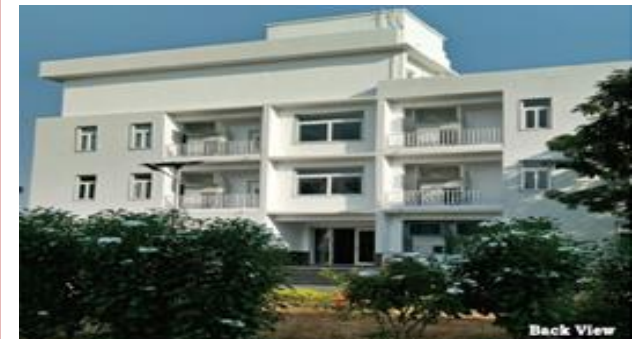
R&E Hub Back View
